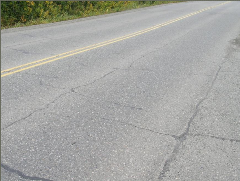
Cracking but stable pavement
