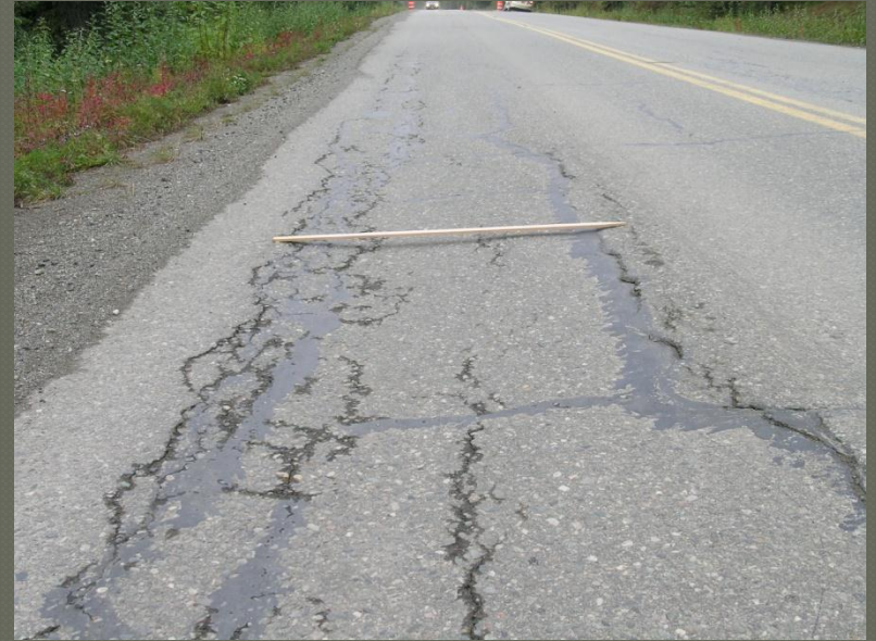
Fatigue and evidence of loss of support
